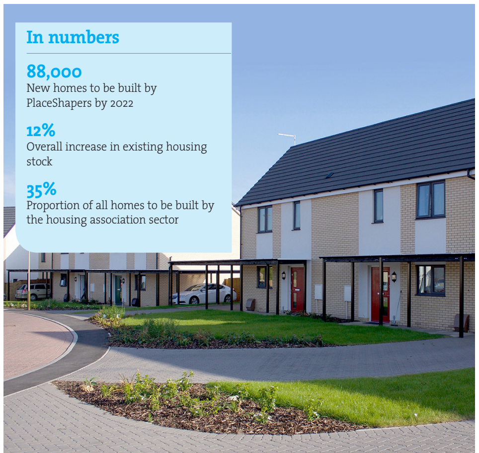
emh group's exemplar scheme of 68 Passivhaus accredited homes in Leicester
