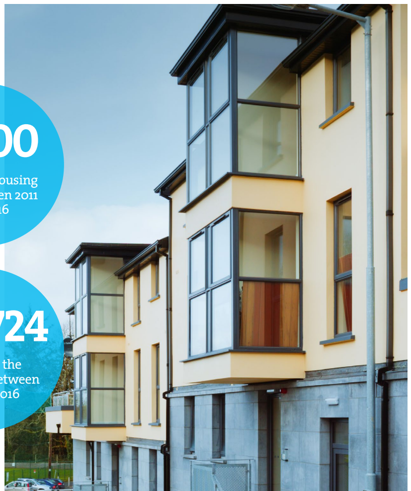
Clúid Housing completed this unfinished apartment block in Macroom in partnership with Cork County Council
